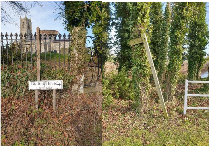
Figure 1, FP7. Post cemented back in place
