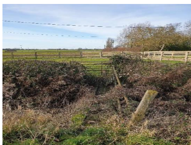
Figure 1, FP9. Bridge rotted and path blocked by fencing. 09/05/2022
